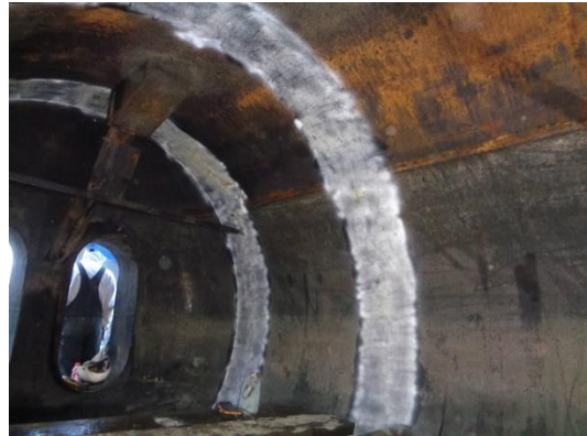
2 x 12" WIDE BANDS WERE MPI AND UT INSPECTED WHERE NEW INLET HORSESHOE DOWNCOMER WAS TO BE WELDED ON SHELL
