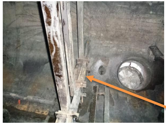
DEFORMATION NOTED ON FIRETUBE BACK SUPPORT BEAM
