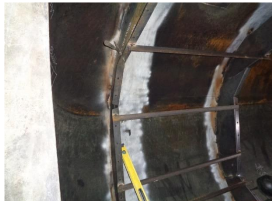
DOWNCOMER TACKED INTO PLACE
