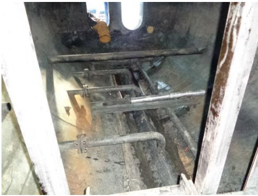
HOT END INTERNALS
