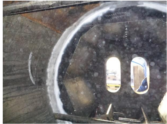
MPI ON FINAL DOWNCOMER TO SHELL FILLET WELD (POST 12HRS) - HORSESHOE PANELS BOLTED IN
