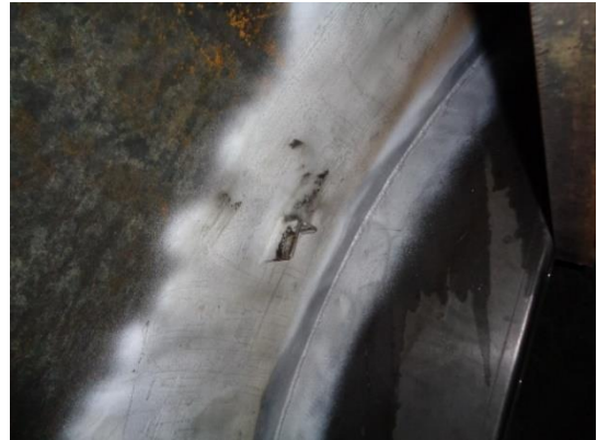
FIRETUBE OVERHEAD DESAND LINE SUPPORT BEAM CUT OFF BUT NOT GROUND FLUSH TO SHELL
