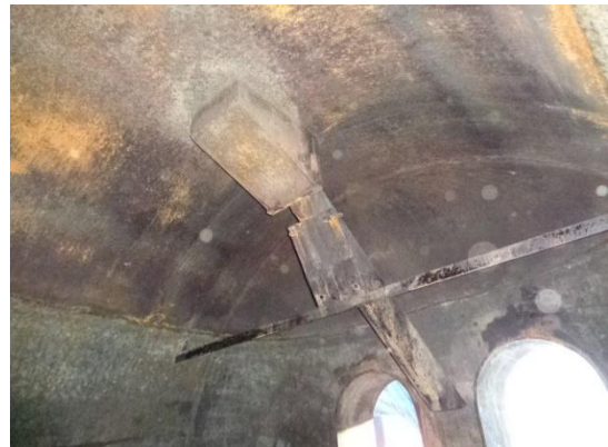
INLET DEFECTOR - WAS REMOVED FOR ADDITION OF INLET HORSESHOE DOWNCOMER
