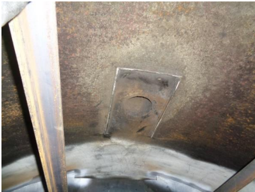
OLD INLET DEFLECTOR CUT OFF BUT NOT GROUND FLUSH TO SHELL
