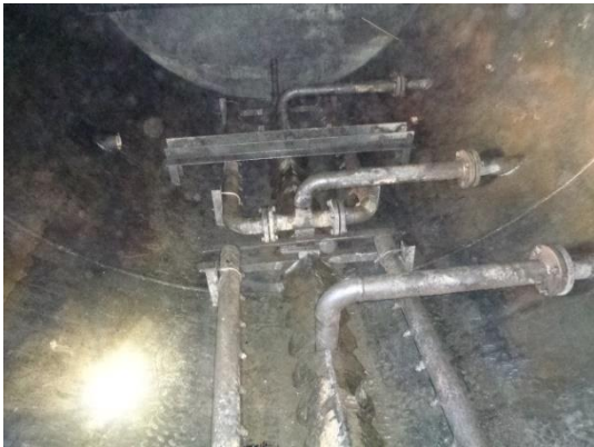
COLD END INTERNALS
