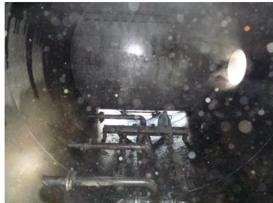
COLD END INTERNAL OVERVIEW LOOKING AT BAFFLE PLATE
