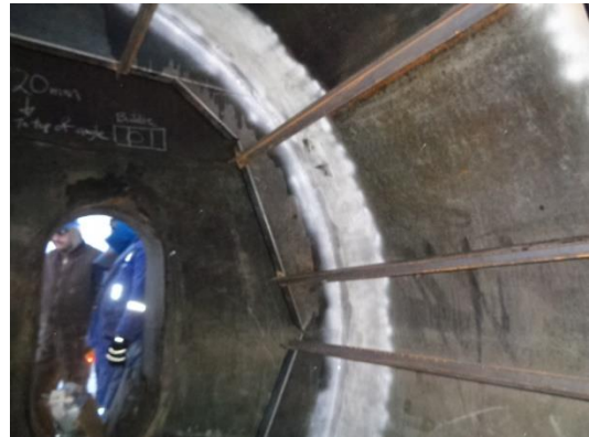
MPI ON FINAL DOWNCOMER TO SHELL FILLET WELD (POST 12HRS)
