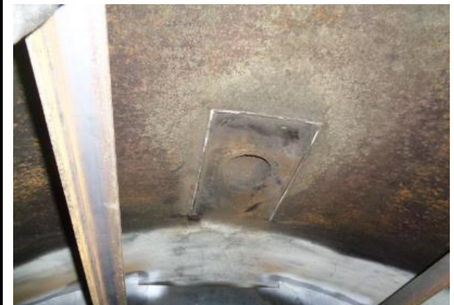
Old inlet deflector box cut off but not ground flush to shell
