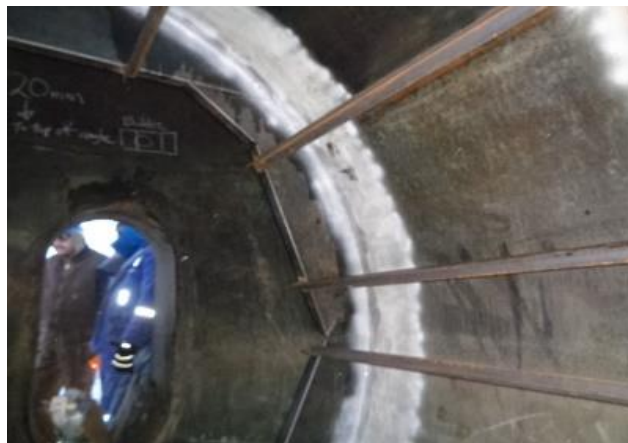
MPI on final inlet horsehoe downcomer to shell fillet welds 12 hours after welding was completed
