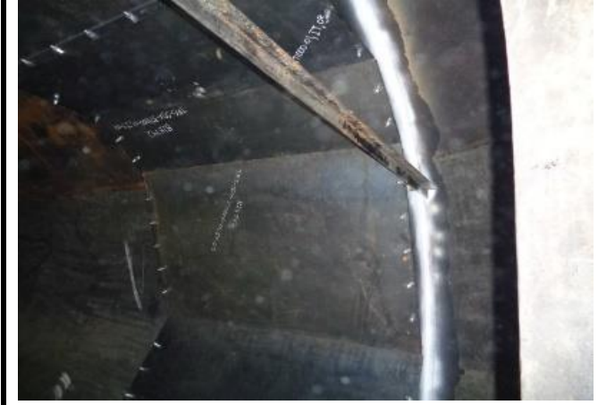
MPI on final inlet horseshoe downcomer to shell fillet welds 12 hours after welding was completed
