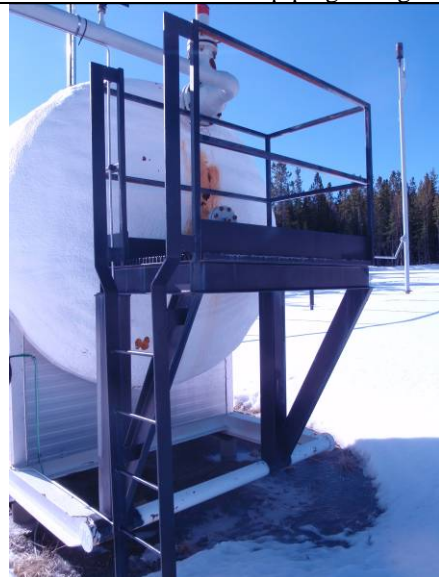
No underside corrosion - Truck-out piping is in good condition.
