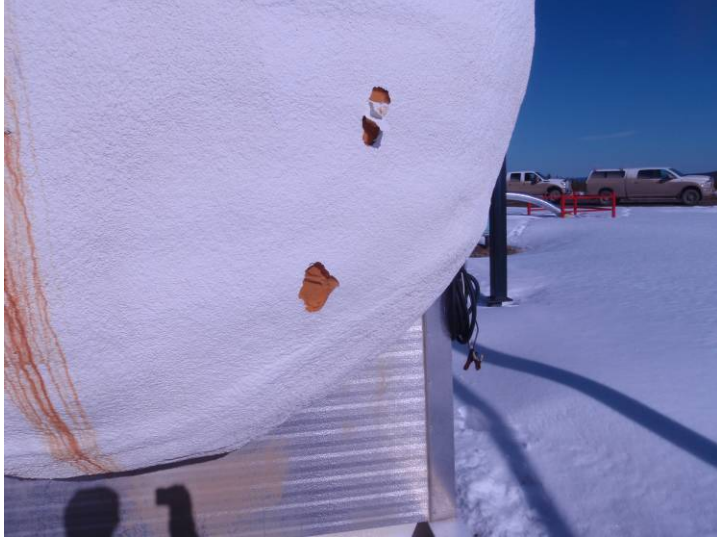
Vessel is welded to the pilings / Ground wire attached
