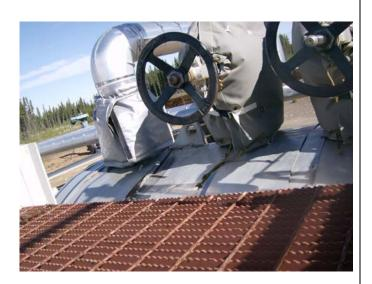
Figure 3\_Insulation damage
