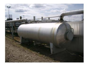
Figure 2\_Flare knockout drum
