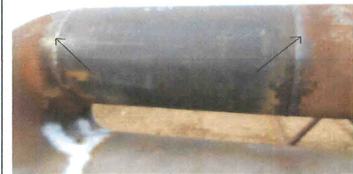
View of 2-butt weld
