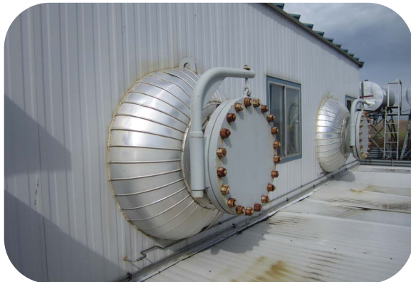
A2864631_North head, Manway and Davit Arm_16July2011
