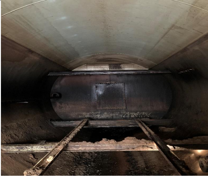
Firetube end picture of internal Weir
