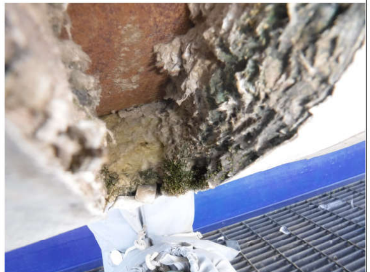
08-Surface corrosion on head and biological growth
