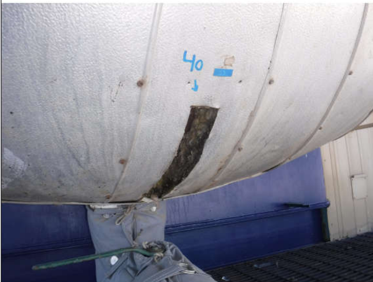
07-Missing insulation covers
