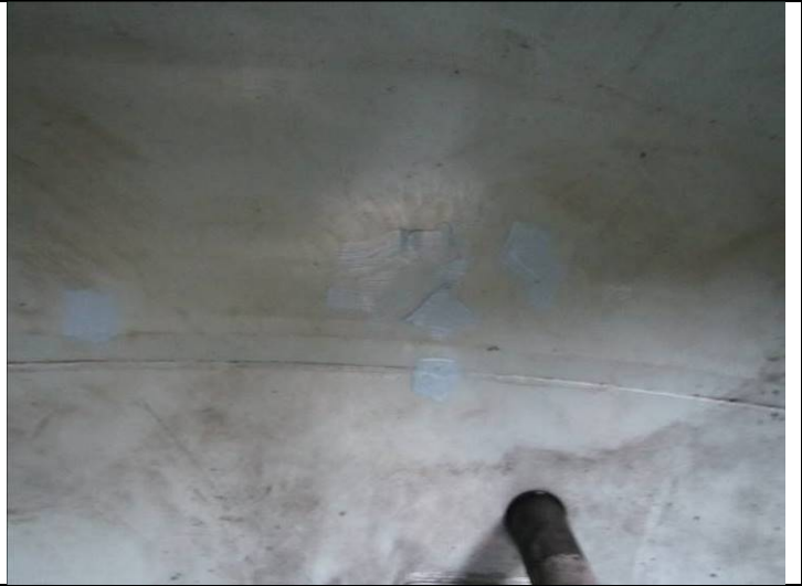
Repairs to coating
