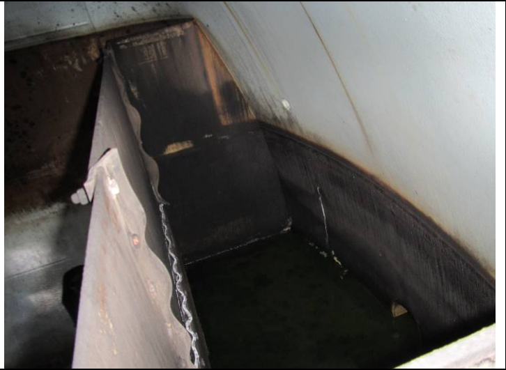
View into spill box
