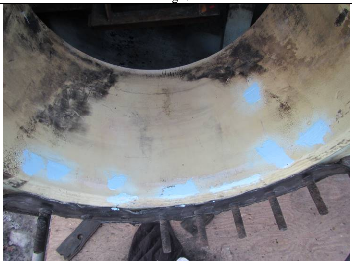
Coating repairs
