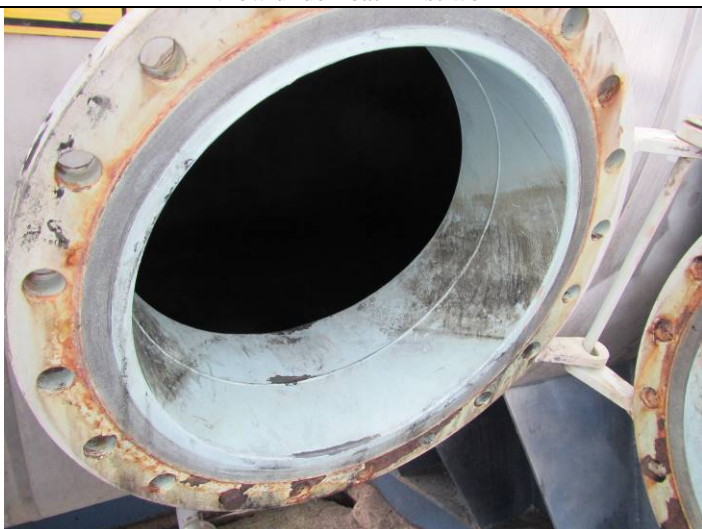
Manway – back end
