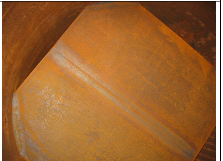
Inlet diffuser plate
