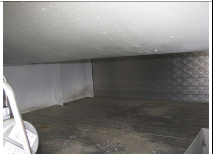
No underside corrosion.
