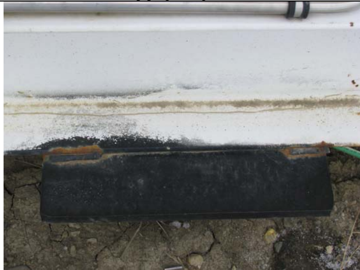
Vessel is welded to the pilings.
