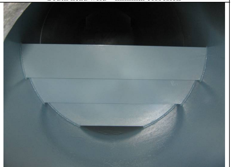
Lower half of vessel internally coated
