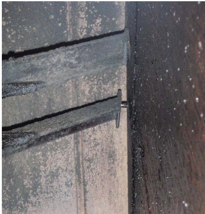
Figure 08_Loose Bolt on Weir Plate Supports
