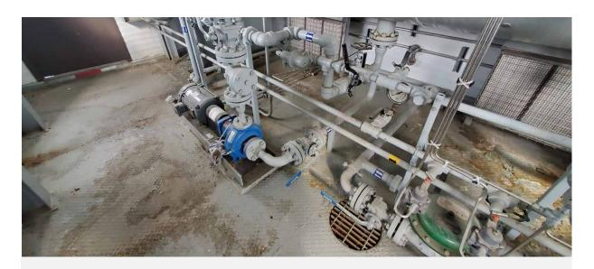
The Goulds pumps were incorporated to help in low pressure applications. The piping is designed so you can either flow through the centrifugal pumps or bypass them completely with no piping changes required.
