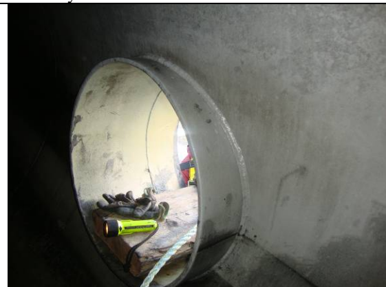
Man way attachment weld coated
