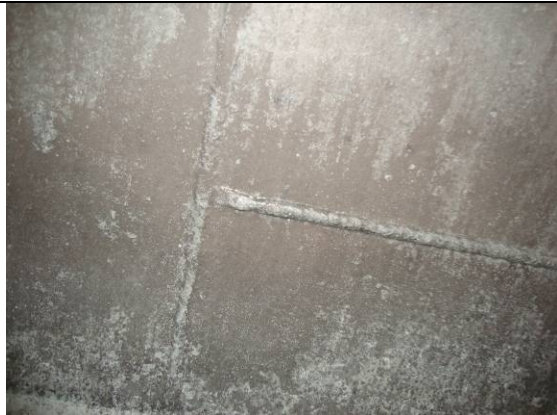
Shell tee weld
