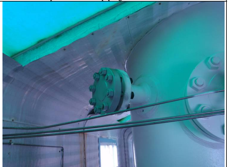
Top head.- Outlet piping and PSV removed
