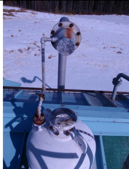
Top head.- Outlet piping and PSV removed
