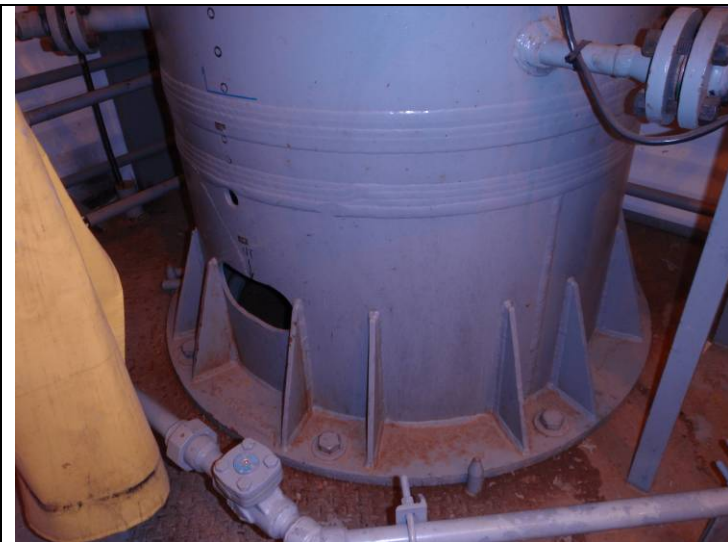
Skirt bolted to skid floor
