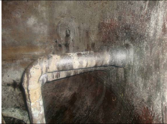
Coil attachment weld to shell
