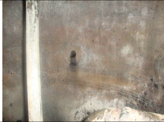
Bottom nozzle and shell to head weld
