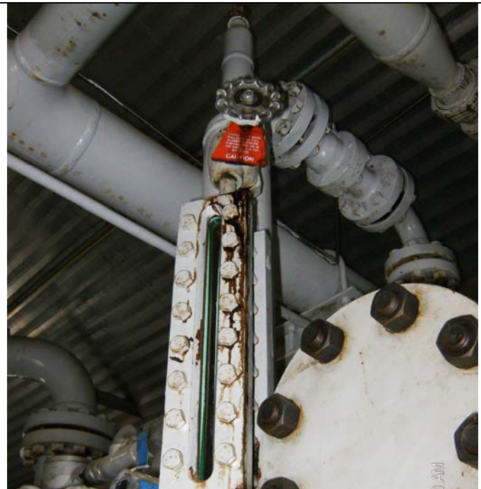
04 evidence of leak from sight glass top packing
