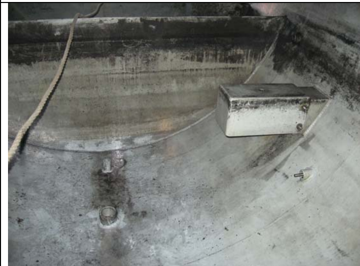
Over view of weir
