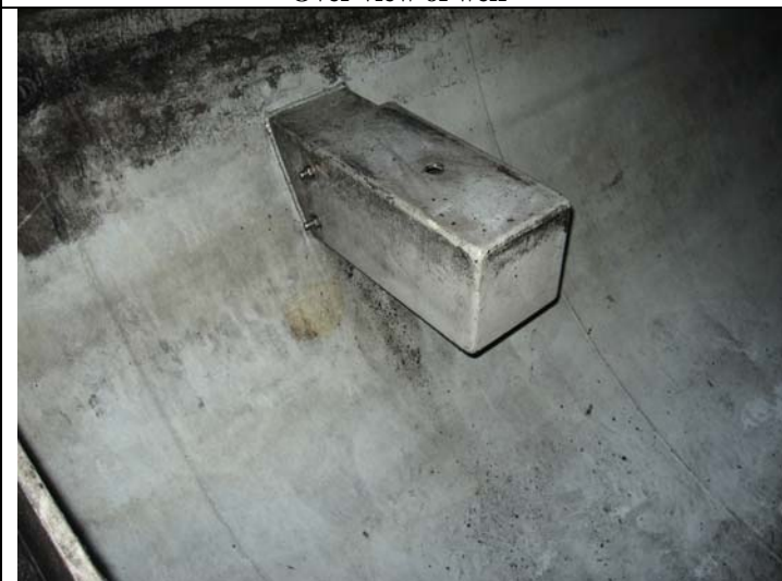
Inlet nozzle diffuser
