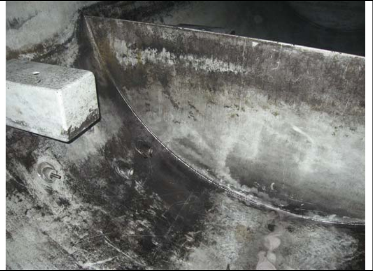
Weir and inlet diffuser
