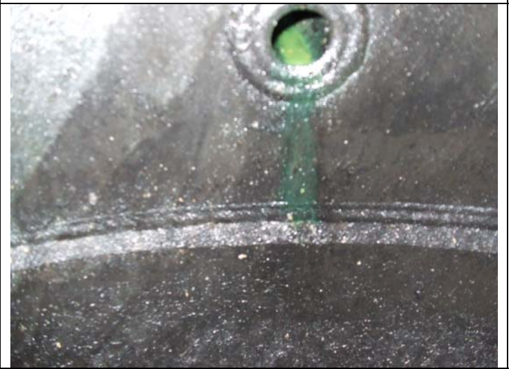
Bottom circ weld Overview
