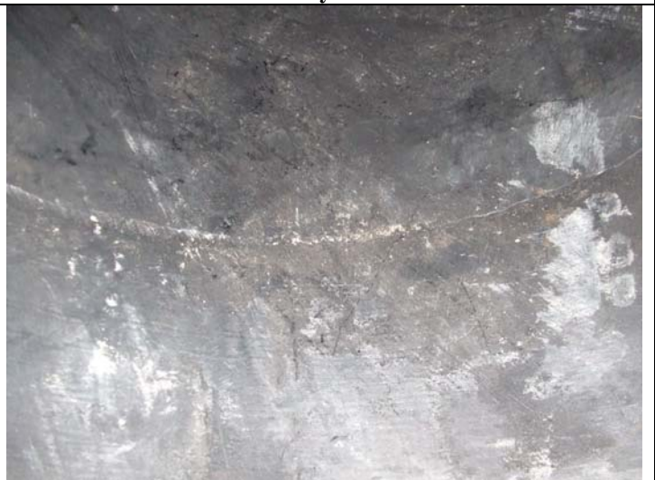
Bottom side of Manway Nozzle
