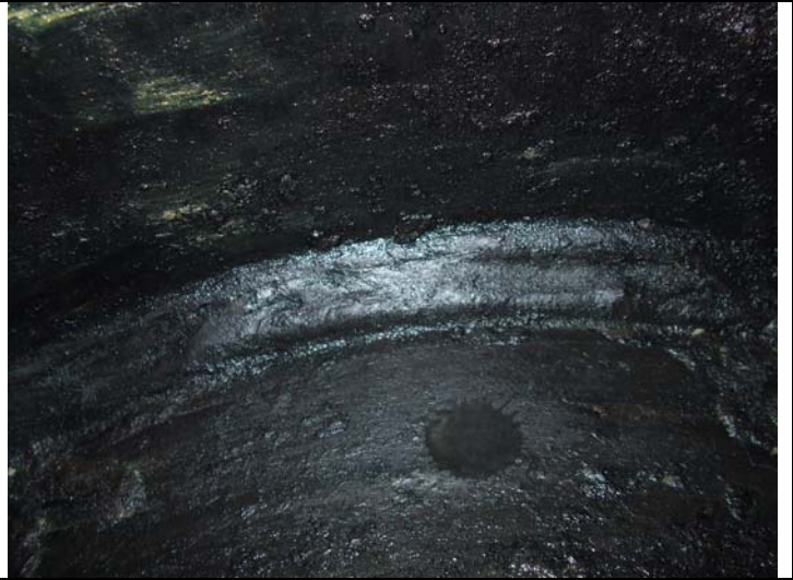
Internal Manway circ weld
