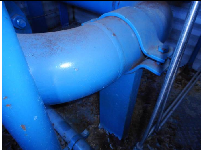
External piping support
