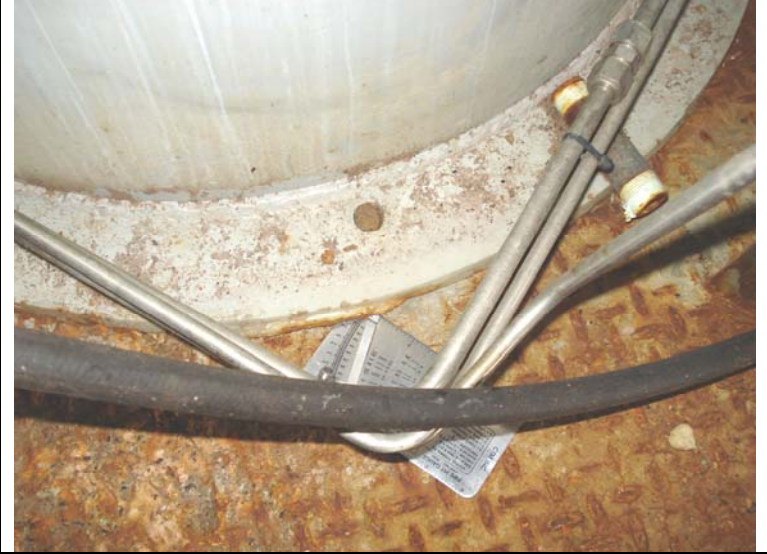
Skirt weld, note not welded.
