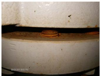
05 paint deterioration with surface scale
