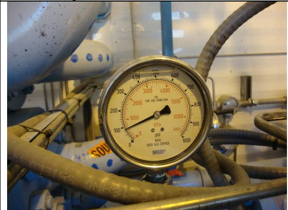
Vessel tube pressure gauge
