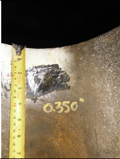
Pit excavated to 0.350 inch depth
