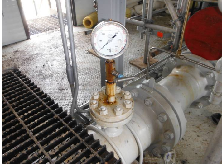
Liquid seepage at pressure gauge valve
