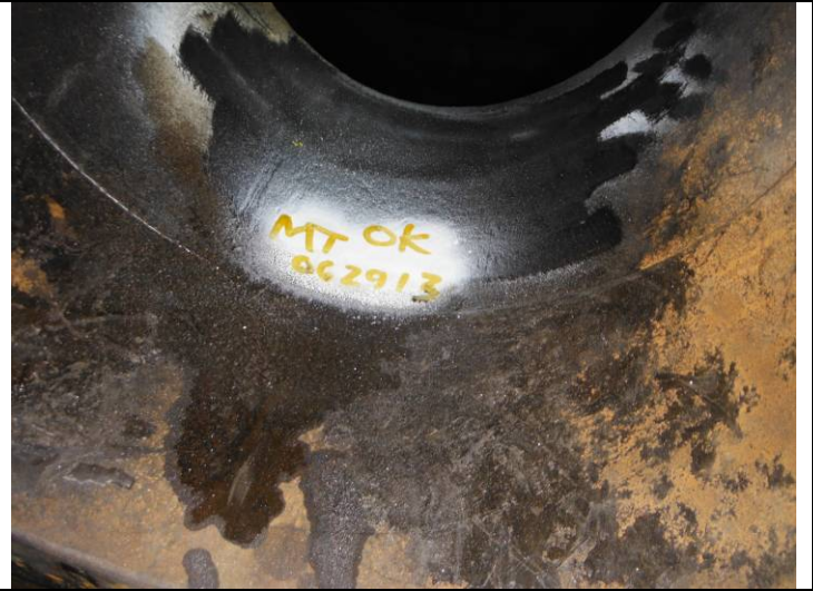
Final repair MT carried out – No cracking detected.
